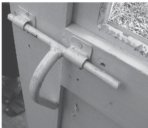
Figure 5.6 Large door bolt, easy to grasp
