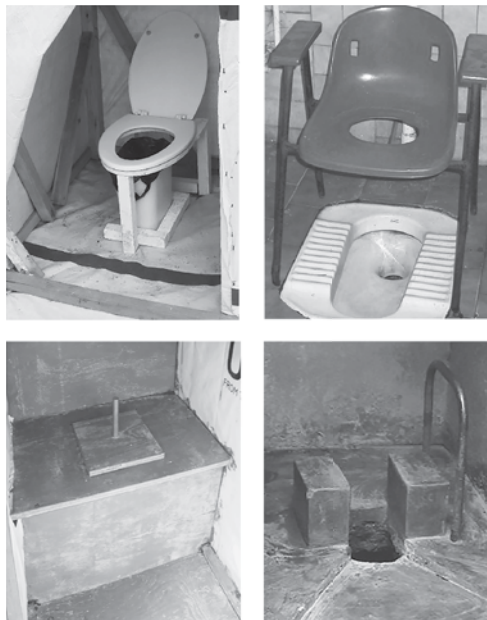
Figure 5.12 Dry pedestal interfaces
